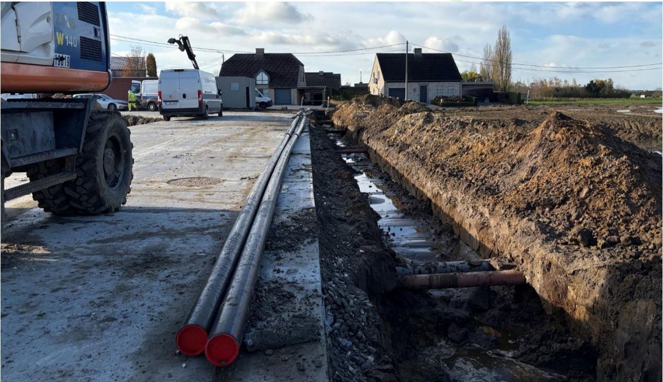
Figure 12: realisation of the secondary circuit on the site
