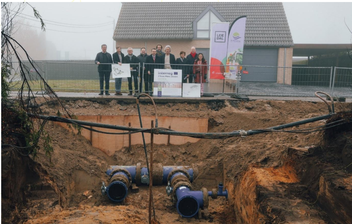
Figure 10: the realisation of the bypass of the drinking water pipe
