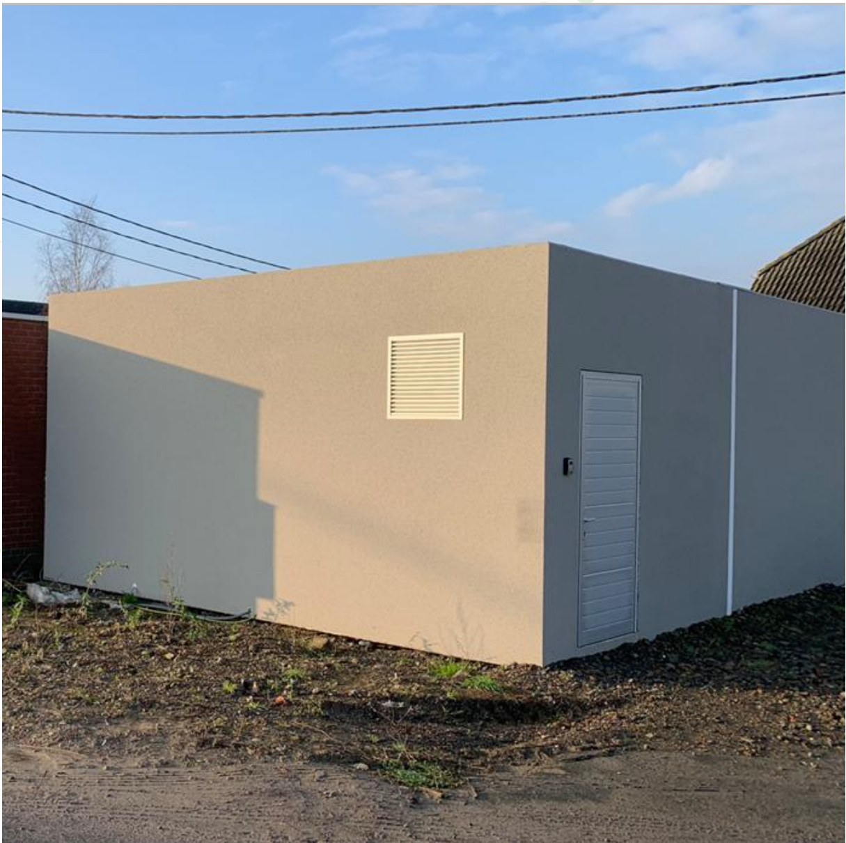
Figure 11: the technical cabin
